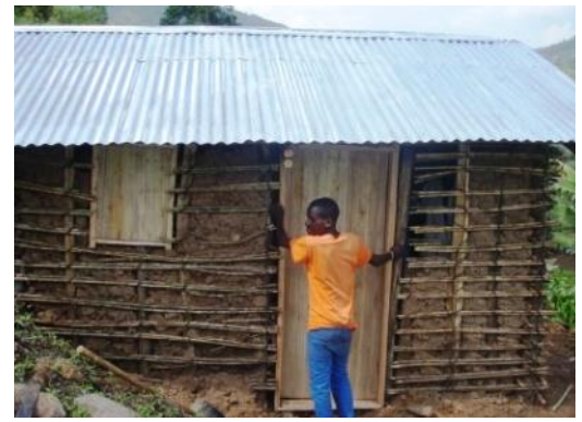
A door is placed on Nossi and Moses's new home.
