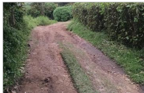
Newly repaired driveway
